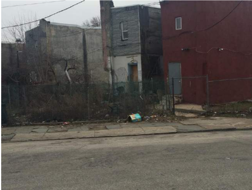
Housing stock is abandoned and in disrepair
